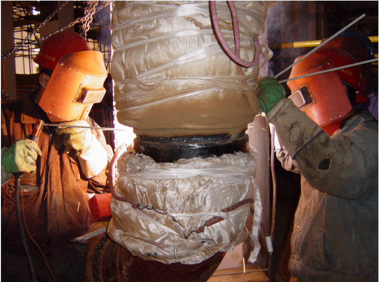
Figure 1 Welding P36 feedwater piping using 1NiMo.B electrodes
