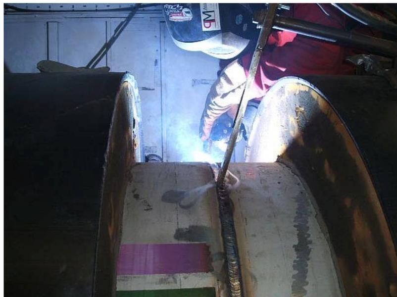
**Figure 12 Gas shielded flux cored arc welding, Supercore 308LCF, being used for the first time during construction of the Grain-LNG importation facility on the Isle of Grain, UK Photograph courtesy of P M Associates UK Ltd**
