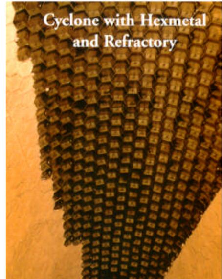
**Figure 4: Detail of cyclone showing (a) hexmetal welded in position and (b) partially filled with refractory**
