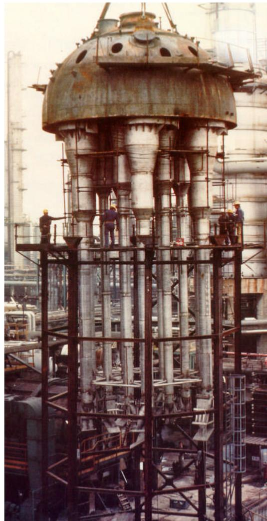
**Figure 3: Regenerator vessel top assembly, complete with cyclones in position**
