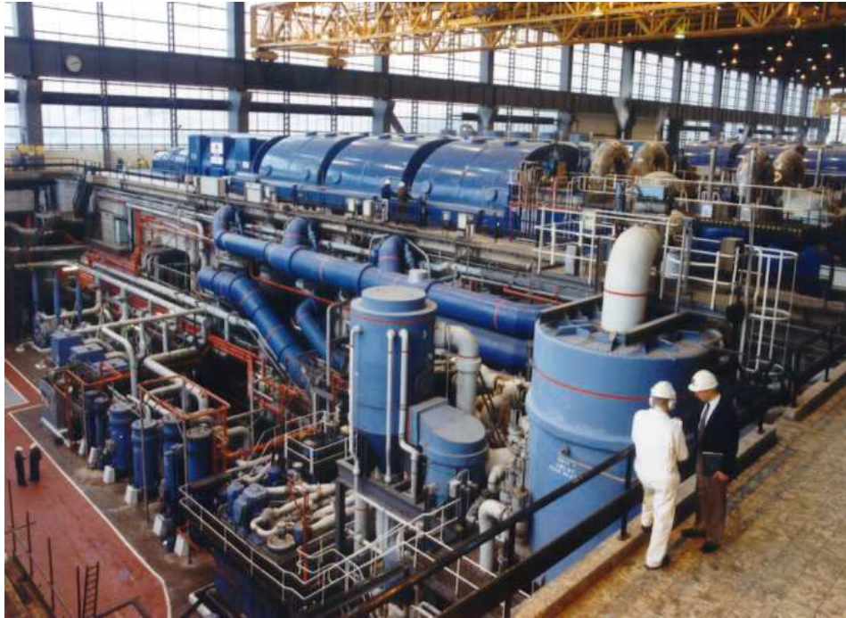
Figure 1 Turbine hall, Eggborough power station, UK
